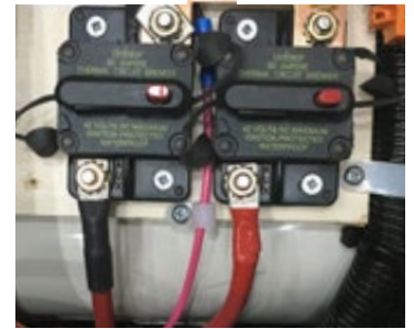
50 AMP BATTERY DISCONNECT BREAKER
